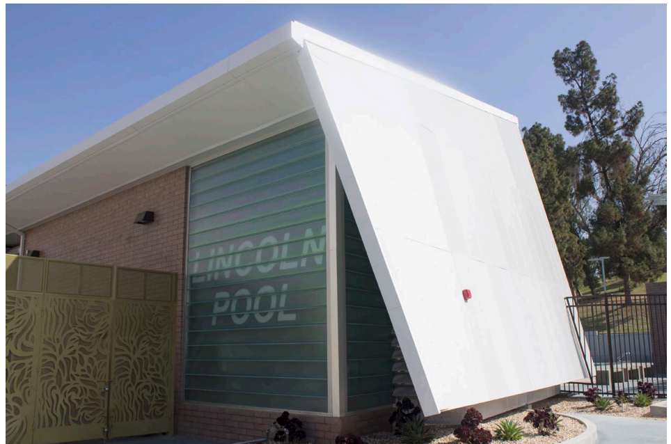
Lincoln Park Recreation Center Pool & Bathhouse Replacement
