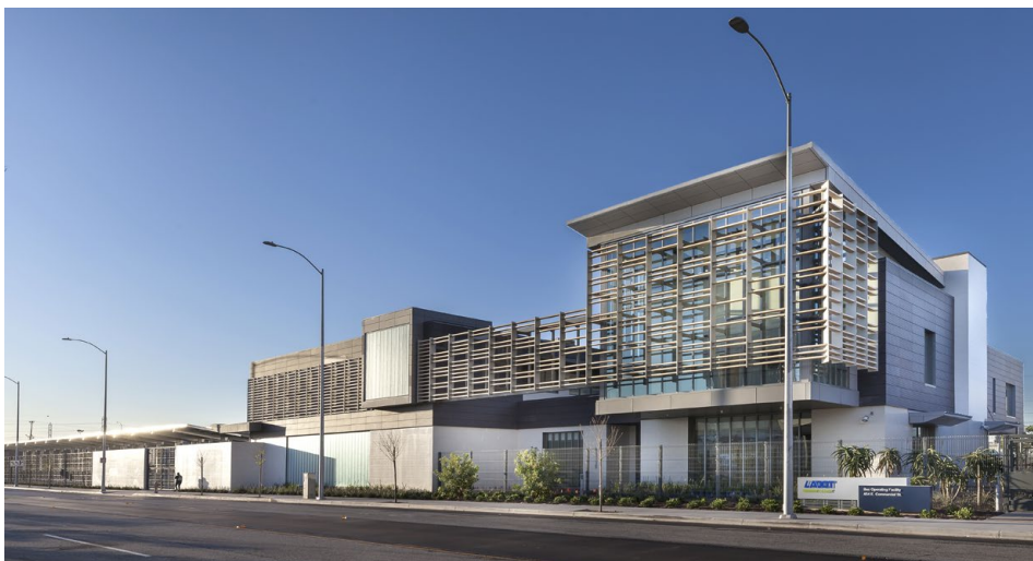
Downtown Bus and Maintenance and Operations Facility
