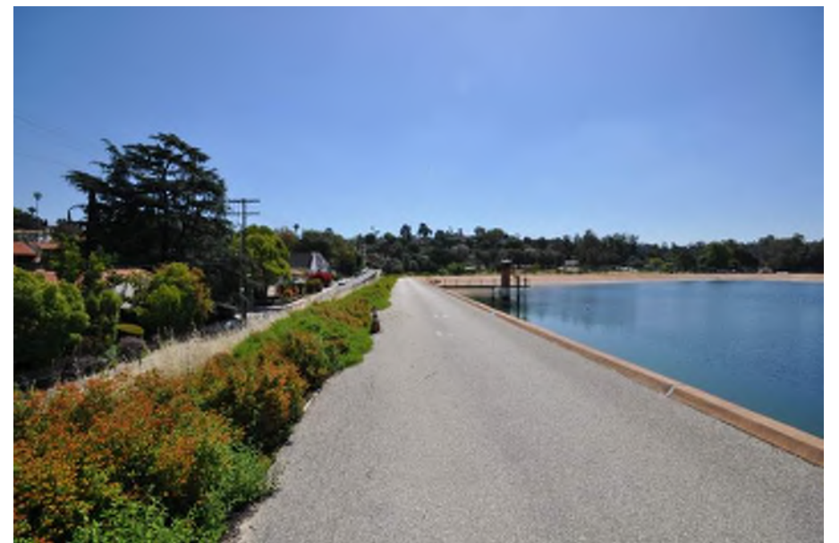
4 North Ivanhoe Dam Chronology: Constructed 1906; altered 1951-53, 1993-94
