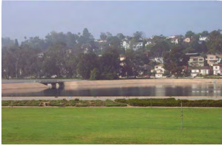
Figure 2-2 Ivanhoe Reservoir and Dam
