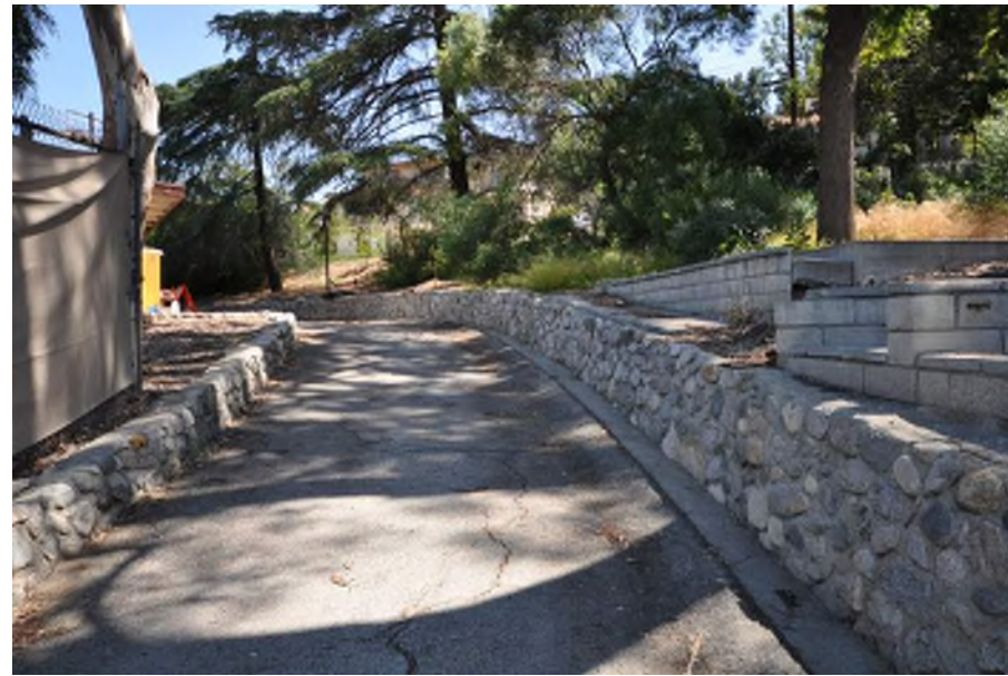
27 Stone Retaining Wall Chronology: Constructed c.1907-10
