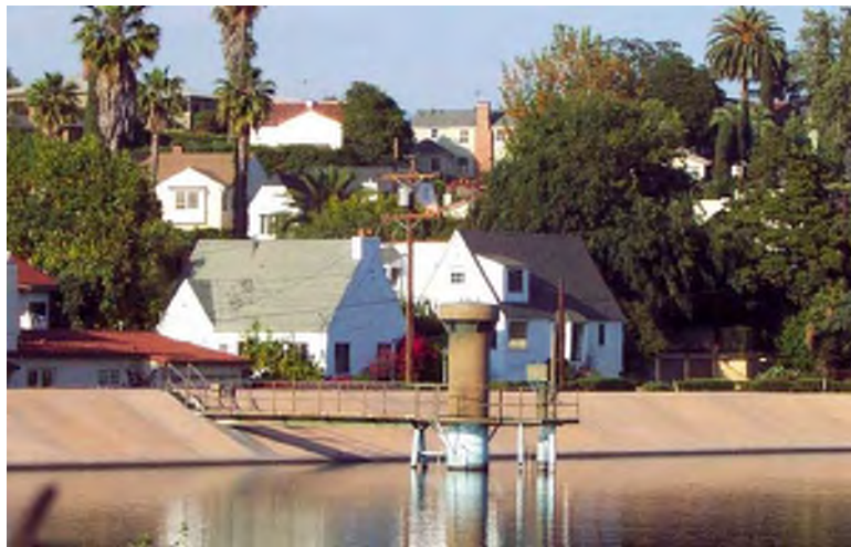
Figure 2-3 Ivanhoe Reservoir Inlet Tower
