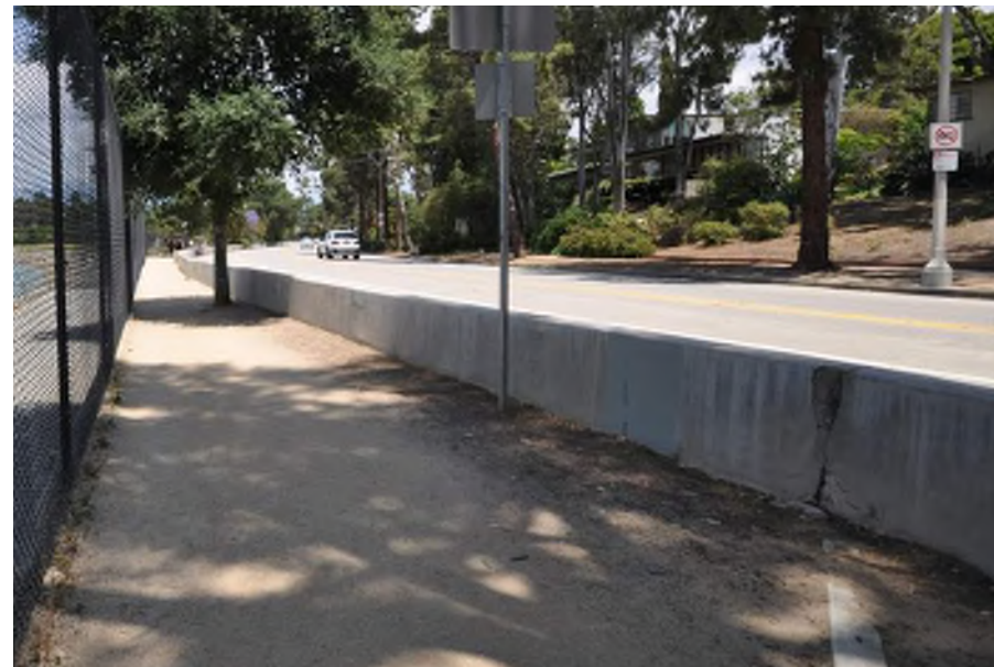
11 Concrete Perimeter Wall Chronology: Constructed c. 1930
