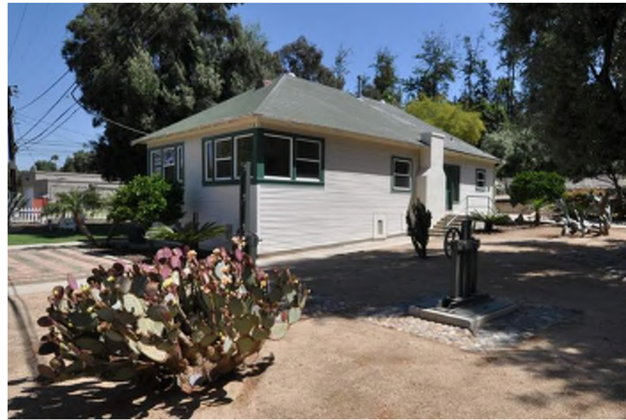
31 Caretaker's House (Sunshine House) Chronology: Constructed c. 1930; altered post-2005
