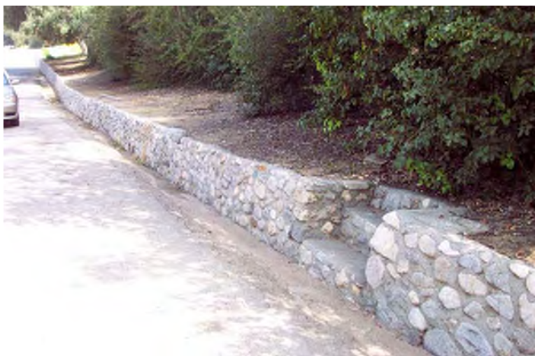
Figure 2-13 Stone Retaining Walls
