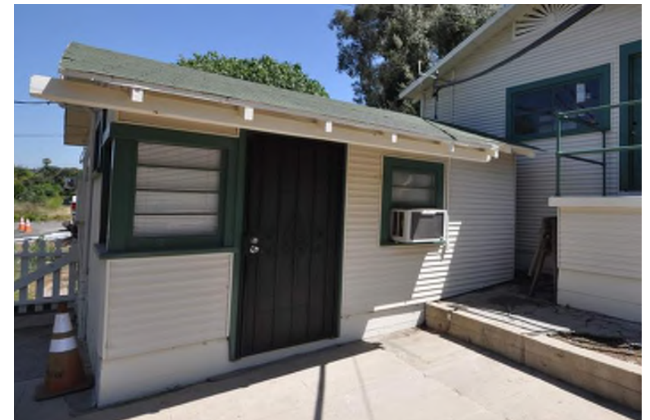
34 Shed (Old Caretaker's House) Chronology: c. 1906-10; altered at unknown date
