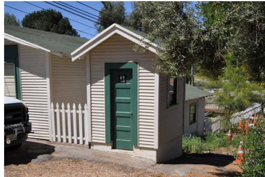
33 Bathroom Building Chronology: Constructed c. 1930; altered post-2005
