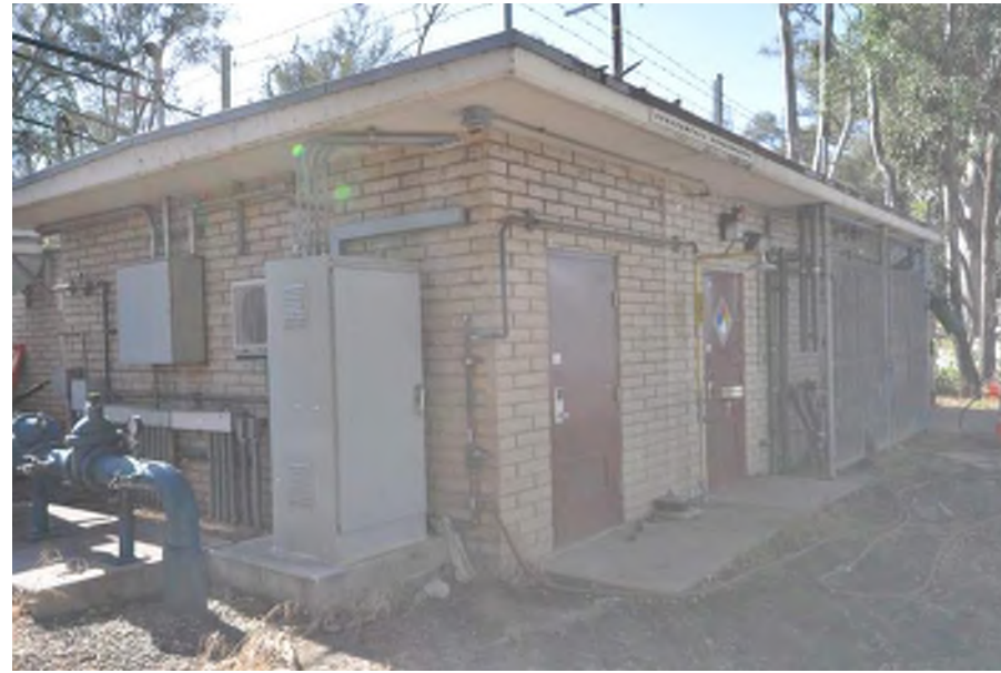
39 Silver Lake Chlorination Building Chronology: Constructed c. 2010
