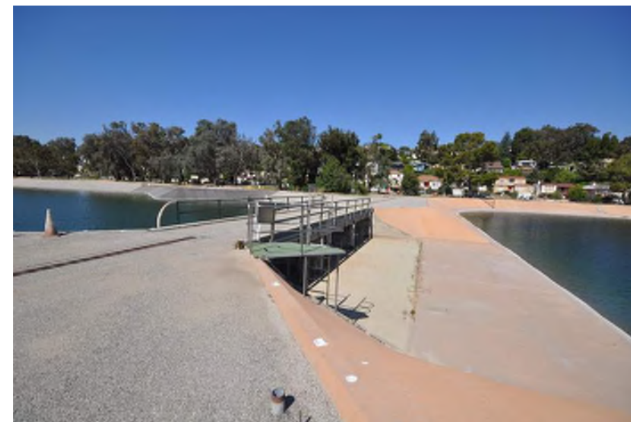
8 South Ivanhoe Dam Chronology: Constructed 1907; altered 1920, 1951-53, 2011-17
