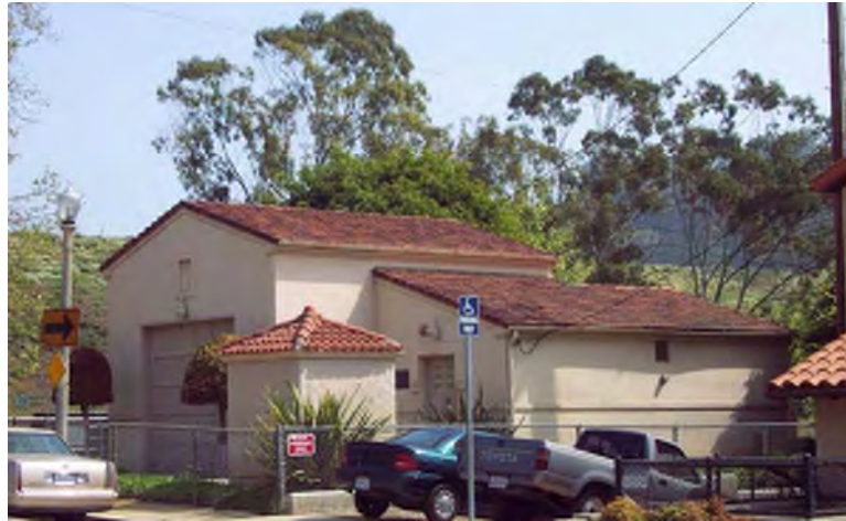
Figure 2-5 Silver Lake South Outlet Chlorination Station and Meter House
