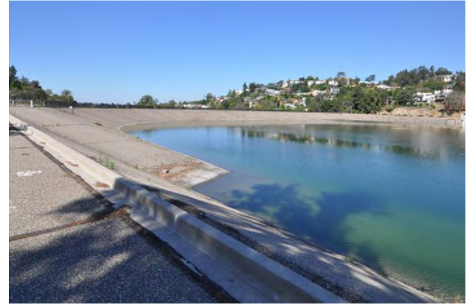
20 Silver Lake Dam Chronology: Constructed 1907; reconstructed 1975-76
