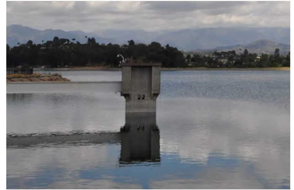
40 Silver Lake Outlet Tower Chronology: Constructed 1937; reconstructed 1975-76
