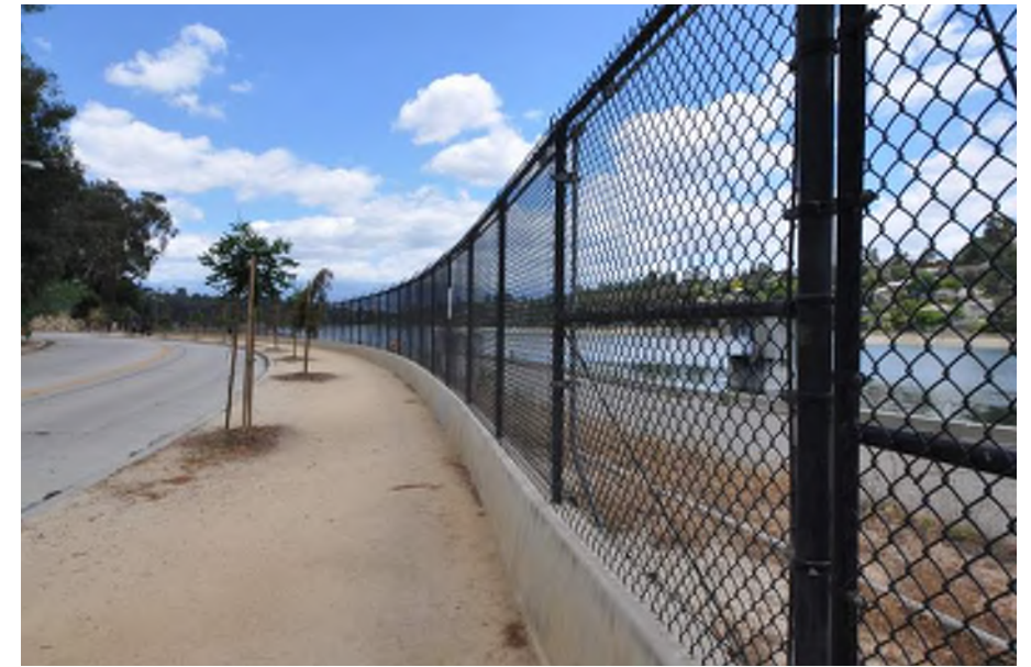
18 West Pedestrian Path, Landscaping, Fencing Chronology: Constructed 2005
