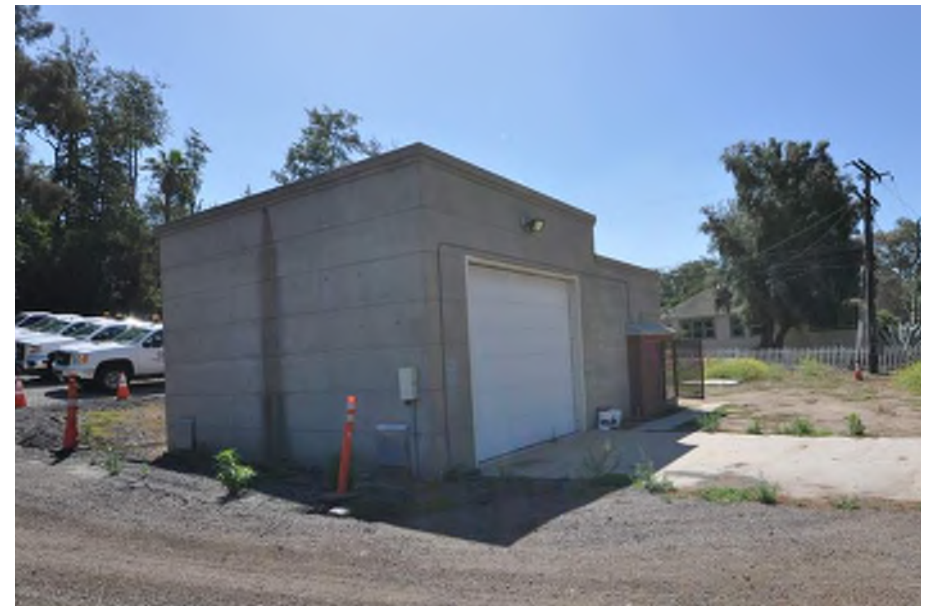
30 Ivanhoe Reservoir Chlorination Station Chronology: Constructed c.1937; altered at unknown date
