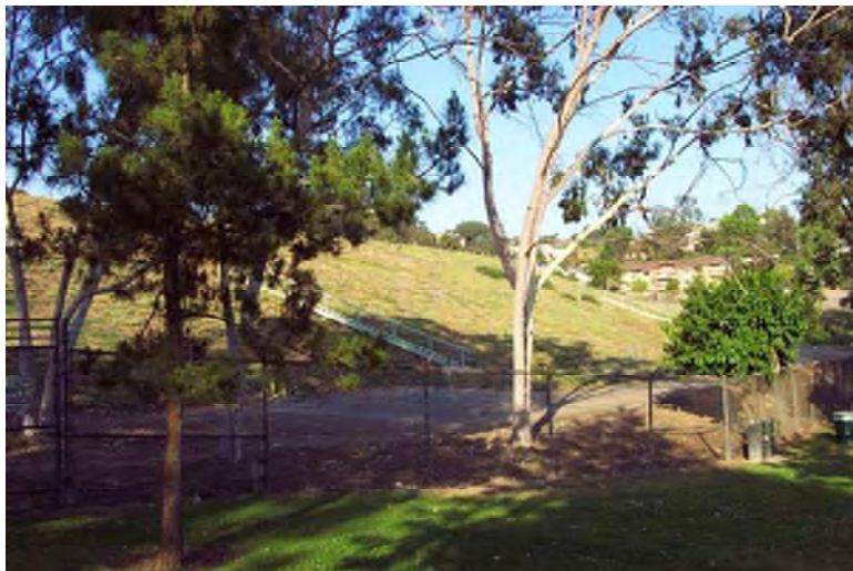
Figure 2-4 Silver Lake Reservoir Dam
