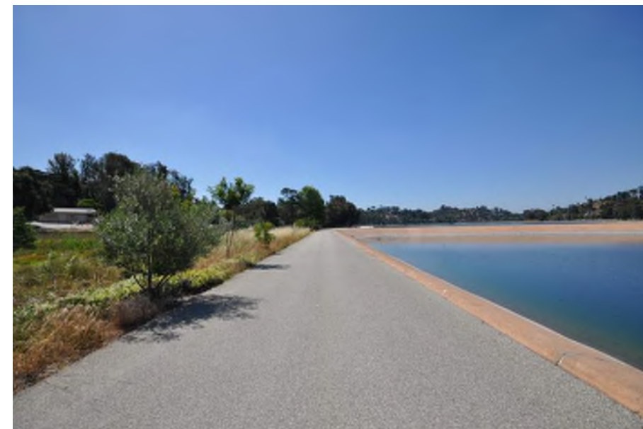
6 Ivanhoe Reservoir Perimeter Path Chronology: Constructed c. 1950
